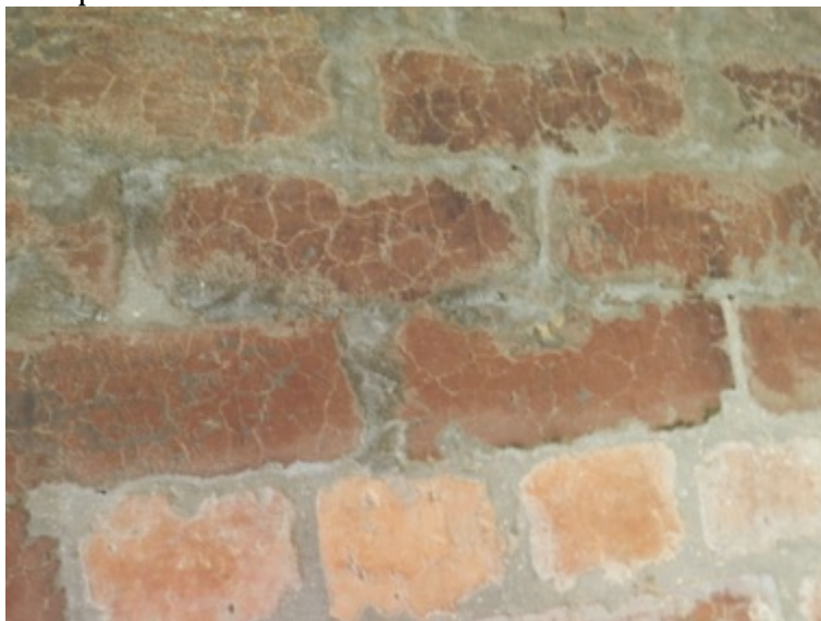
The glazed interior fire-bricks
