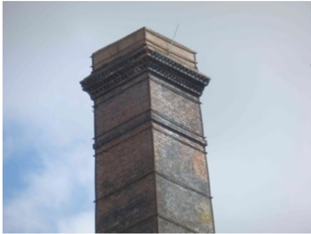
Top and iron bands on a brickworks chimney
