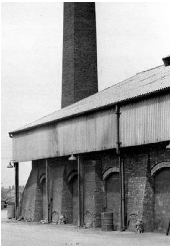
Rectangular kiln and chimney
