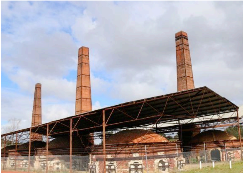
Circular brick kilns and chimneys
